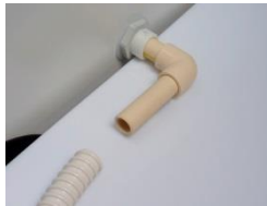
Condensate drain connection with a 90° bend – preparation for sliding-in of the hose
