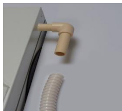
Condensate drain connection with a 90° bend – to slide in the hose
